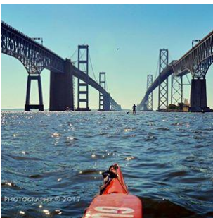
Between the two bridge spans.
